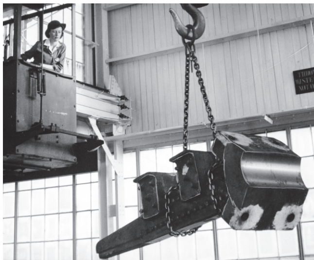
(Above left) 30-ton crane operator at DuPont plant, Wilmington.
